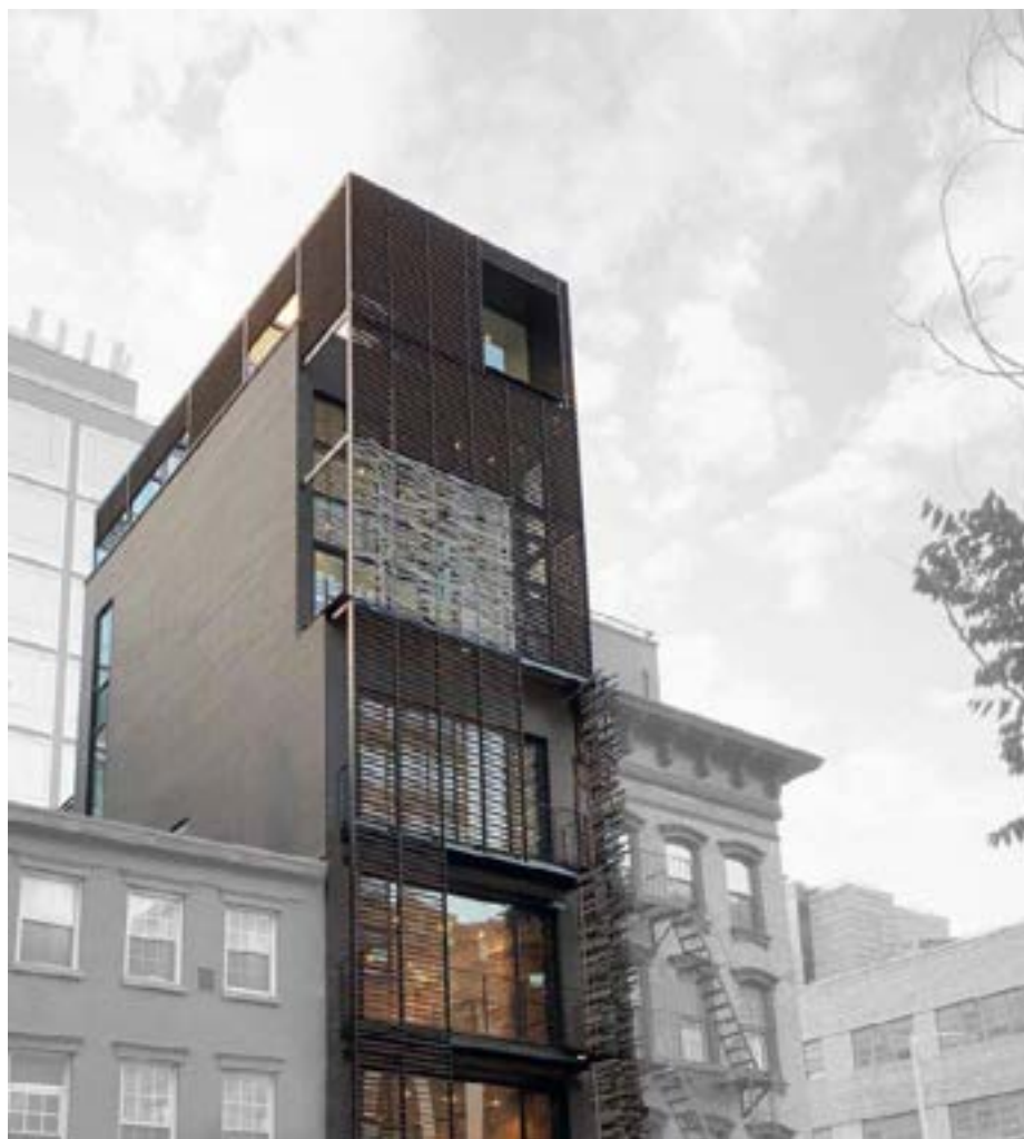
Trellis open (Photo: Archi-Tectonics)
