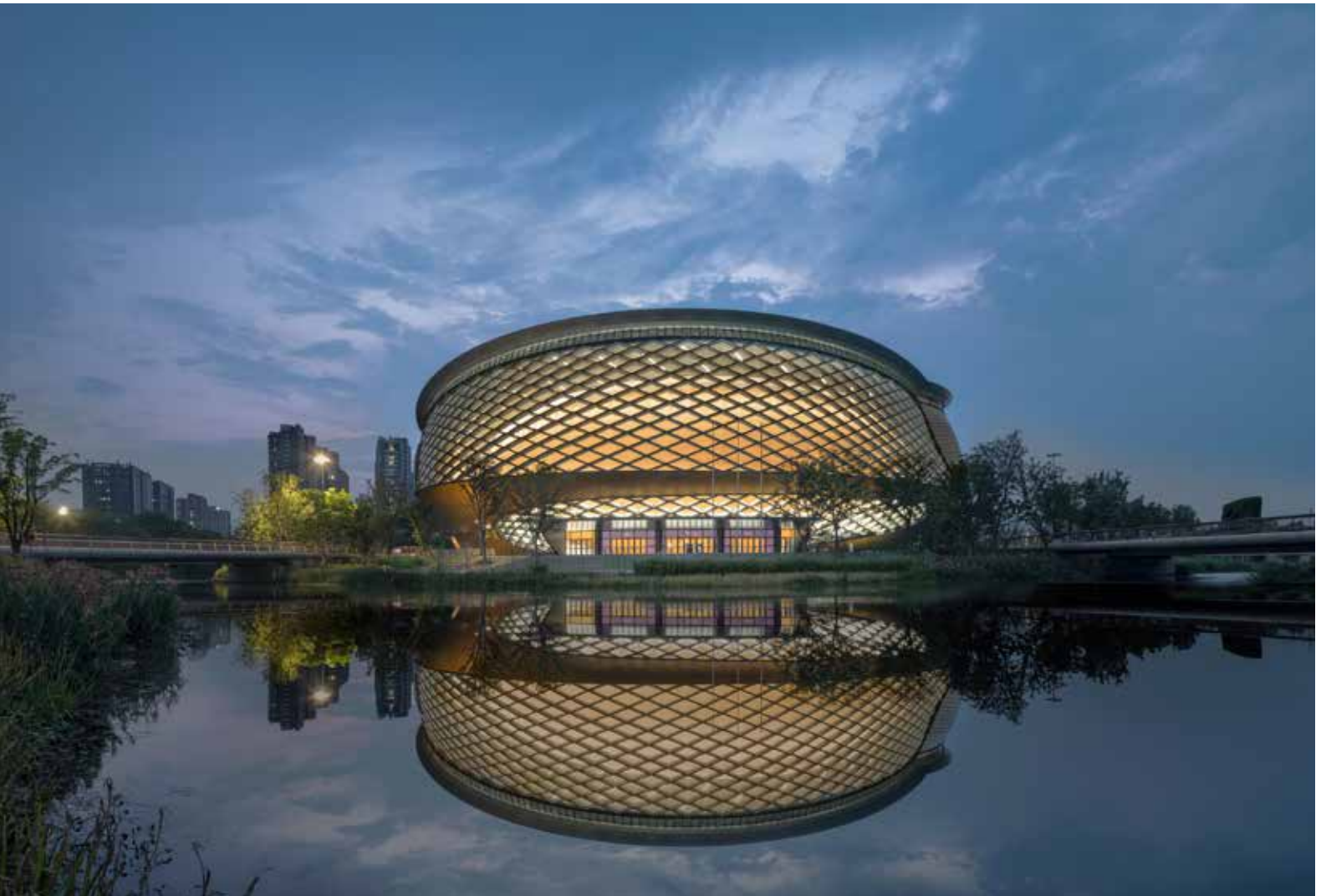
(Above) A night view of Hybrid Stadium flanked by footbridges linking it to two nearby metro stations.
