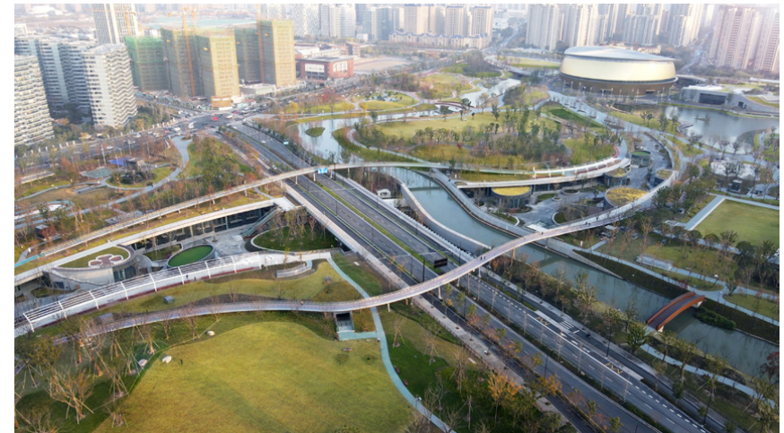
Figure 8.4 Archi-Tectonics, Asian Games, Hangzhou, China, 2022: The site strategy provided by the client was rejected by the design team, favoring one that allowed both a formal and programmatic linkage between two stadiums planned for the site. A green pedestrian valley, with retail spaces on each side traverses the site at the lower level, connecting the stadiums via an outdoor walk and green space with green-roofed glassed façade pavilions and long solar-paneled wings that shade visitors.
