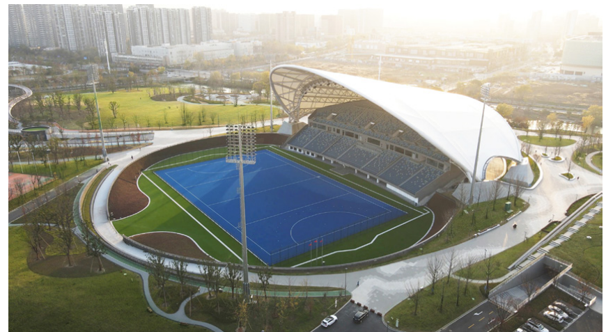
Figure 8.14 Archi-Tectonics, Asian Games, Hangzhou, China, 2022: The 125-meter roof span of the field hockey stadium is dramatic, and covers the entire spectator seating area, which is organized on one side of the playing field. The field itself is set 5 meters into the ground to further blur the relationship of landscape and the structure, and contains large concrete abutments to anchor the large span roof.
