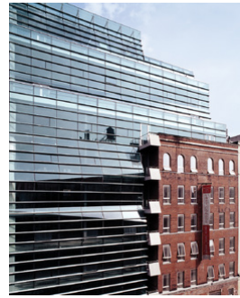
Figure 8.2 Archi-Tectonics, Greenwich Street Building, New York, NY, 2000. Folded double glazing with a solar film allows the glass façade to perform specifically for the New York climate. The glazing allows for solar penetration from the low winter sun, providing passive solar energy, while the solar film protects from the harsher summer sun, removing solar glare. Such an example of form-as-performance, articulated by Manuel DeLanda and others, was an early goal of architects engaging the digital.
